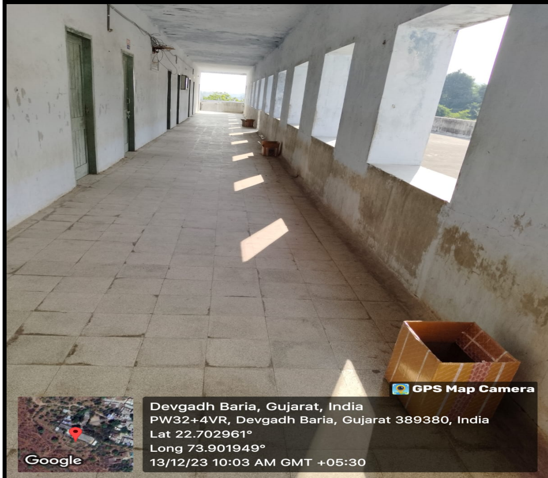
Daylight in Corridor Area
